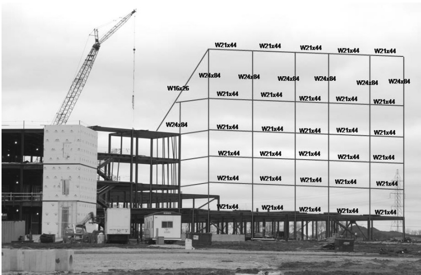
Figure 6. A conceptual image of AR overlay of 3D design and contextual data.
